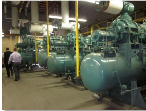
Cold storage and blast freeze plant, Port of Los Angeles, Terminal Island Land Use Plan, LWC
